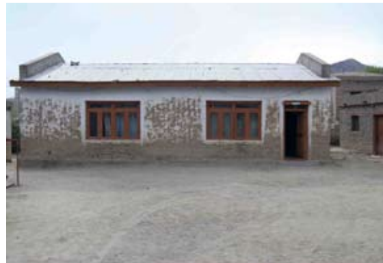
Library building after repairs.
