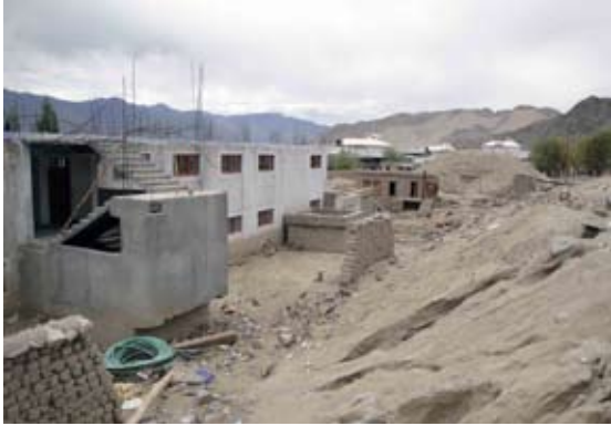
Leh hostel compound wall before repairs.
