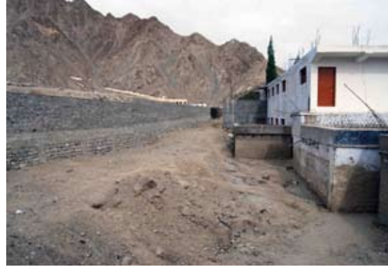
Leh hostel compound wall after repairs.
